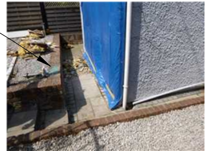
No visible damage to render in this location, but will require replacement across entire elevation in order to achieve a waterproof envelope and acceptable visual appearance. Any junctions with existing render should be cut flush and provided with a sealed movement joint with a drip detail.
